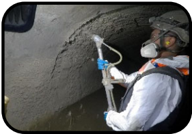
4. Shotcrete Application of Mortar
